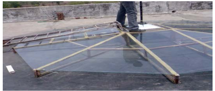
Fig. 2. Experimental setup of solar chimney
