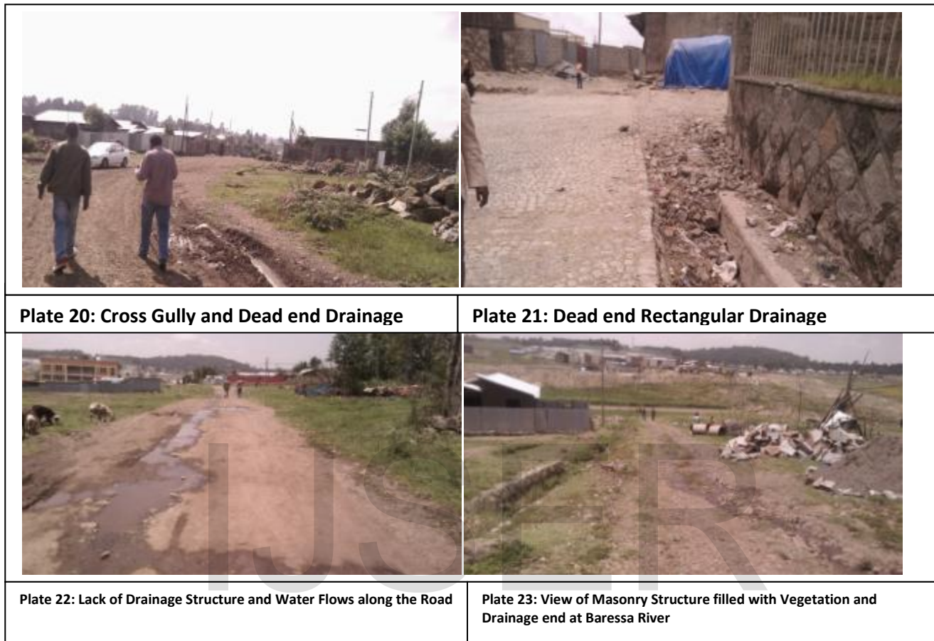
Figure 6. 6Conditions of Drainage Structure
