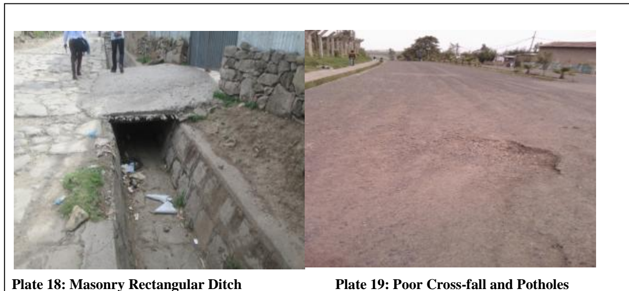
Figure 6. 5Masonry Ditch and Potholes
