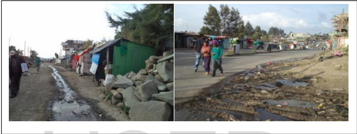
Figure 6. 4Views of Poor Drainage Network (Lack of Road Side Drainage Structure)
