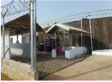
Figure 3. Holding retention tank at Fiamah treatment plant
