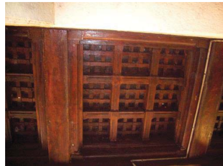
Fig 17 Ceiling of Gopura after Renovation
