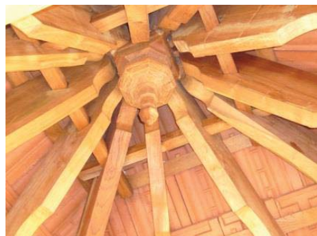
Fig 14 New Jala fixed to the old rafter
