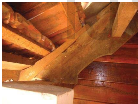
Fig 14 New Jala fixed to the old rafter
