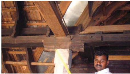
Fig 12 Decayed Beams being Replaced with New
