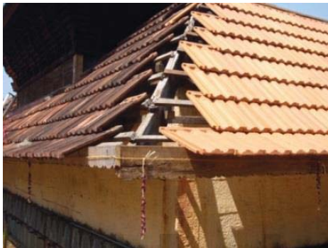
Fig 13 Old Tiles replaced with new
