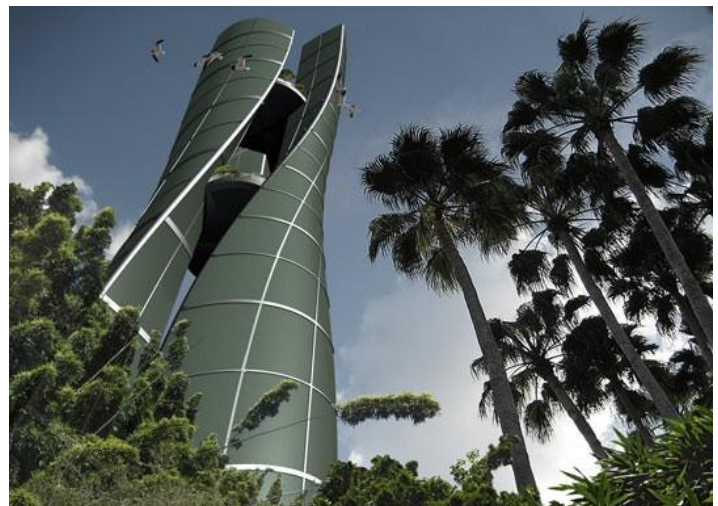
(13) Wind Turbine Tower
