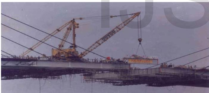
Figure 4. The mid-portion of the deck of the Second Hooghly Bridge being constructed, vividly showing some of the high capacity cranes used.
