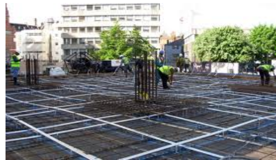
Fig.4 post tensioned flat slab
