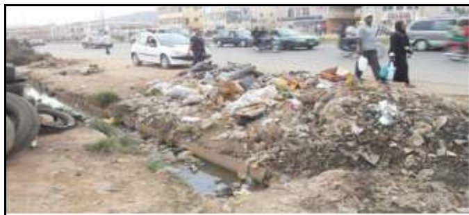
Fig. 4. Mixed Solid Wastes Removed from Drainage Channel on Abacha Road [24].
