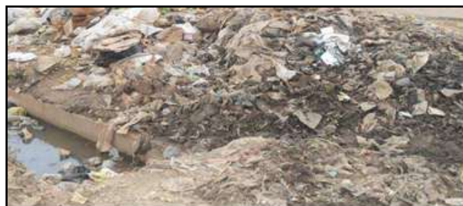
Fig. 3. Mixed Solid Waste Cleared from Drainage Channel on Abuja-Keffi Expressway
