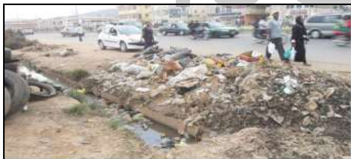
Fig. 5. Mixed Solid Wastes Removed from Drainage Channel on Abacha Road [24].
