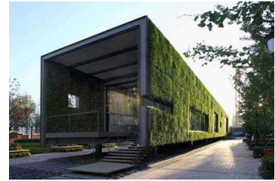
Figure 1.10: Green Nanoarchitecture Source:[ http://beccysoc.webs.com/Retrieved September, 2011-09-01]
