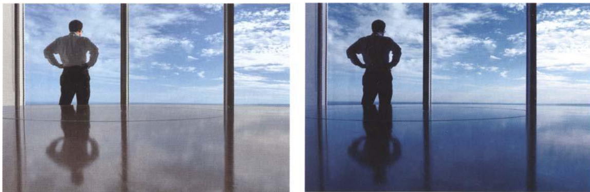
Figure 4.33: Electrochromic glass with an ultra-thin nanocoating needs only be switched once to change state, gradually changing to a darkened yet transparent state. At present the maximum dimension of glazing panels is limited.
