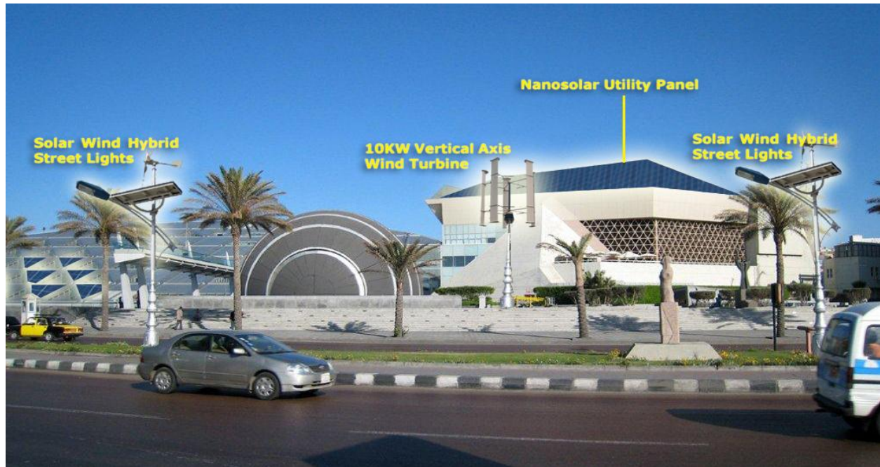
Figure 4.27: External Elements of renewable energy sources in plaza of Bibliotheca Alexandrina.
