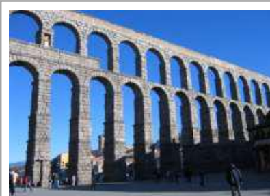
Figure 1.88: The Roman use of the arch and their improvements in the use of concrete facilitated the building of the many aqueducts throughout the empire, such as the magnificent Aqueduct of Segovia and the eleven aqueducts in Rome itself.
