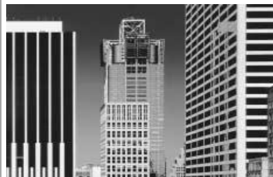
Figure 2.78: The Four Times Square Building in New York City uses thin-film PV panels to reduce the building's power load from the utility grid.
