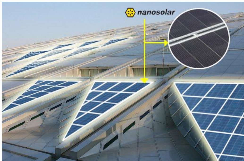
Figure 4.28: Nanosolar Cell on roof of Bibliotheca Alexandrina ( Suggestion places )
