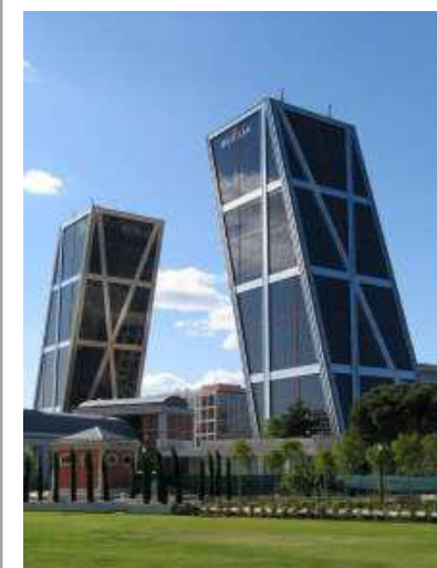
Figure 1.90: Europe's Gate, Madrid; the first intentionally inclined buildings in the world designed by Philip Johnson and John Burgee and commission in 1996. Source: [http://www.recoveryinsulation.co.uk/energy.html, Retrieved September, 2011-
