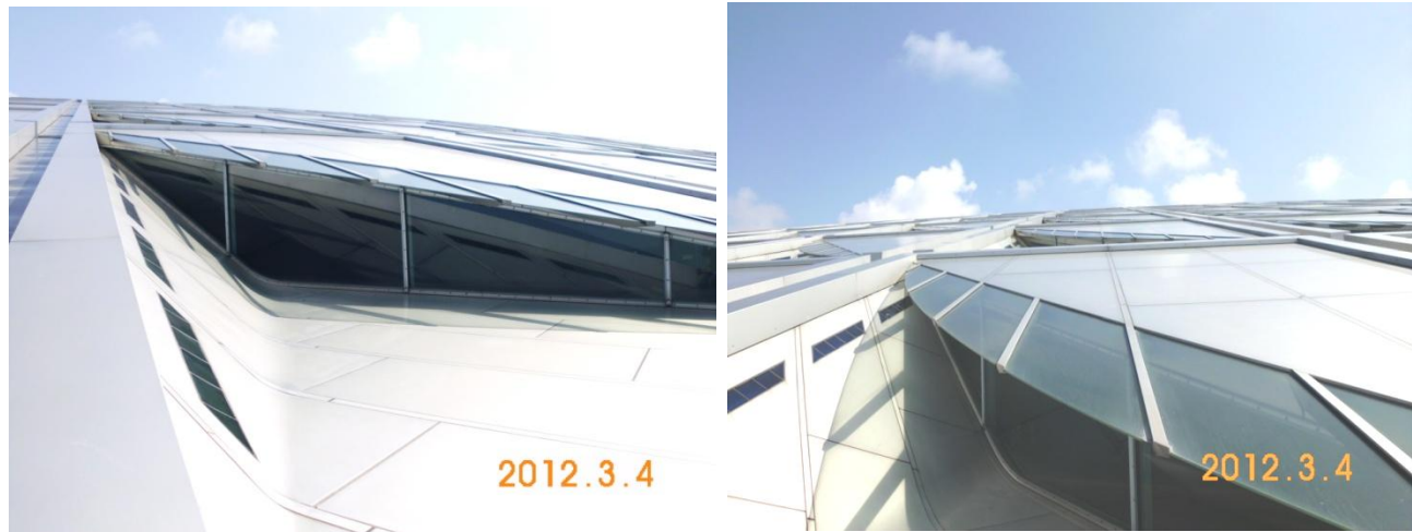
Figure 4.12: Vertical glass rooflight (external view)
