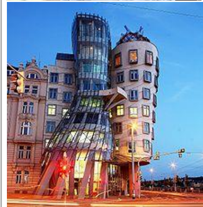
Figure 3.16: Frank Gehry and Dancing House in Prague example for his work. Source is http://en.wikipedia.org/wiki/Frank_Gehry , Retrieved 12 November, 2011]
