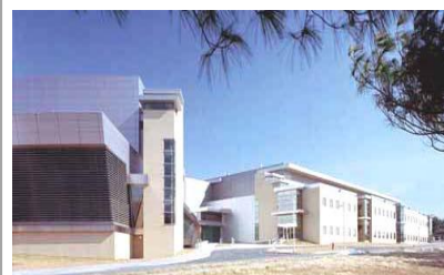
Figure 3.42: The National Institute of Standards and Technology (NIST) Advanced Measurement Laboratory was designed by HDR Architecture Inc. Gaithersburg, Maryland. [Source is http://www.help-stop-globalwarming.com/global-warming-recycling.html , Retrieved 20 November, 2011]
