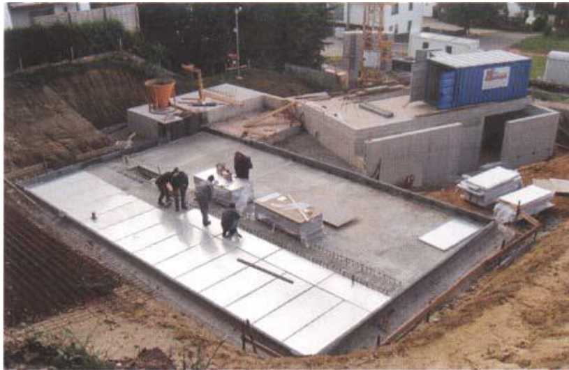
Figure 4.30: VIP insulation must be made to measure and fitted precisely on site.
