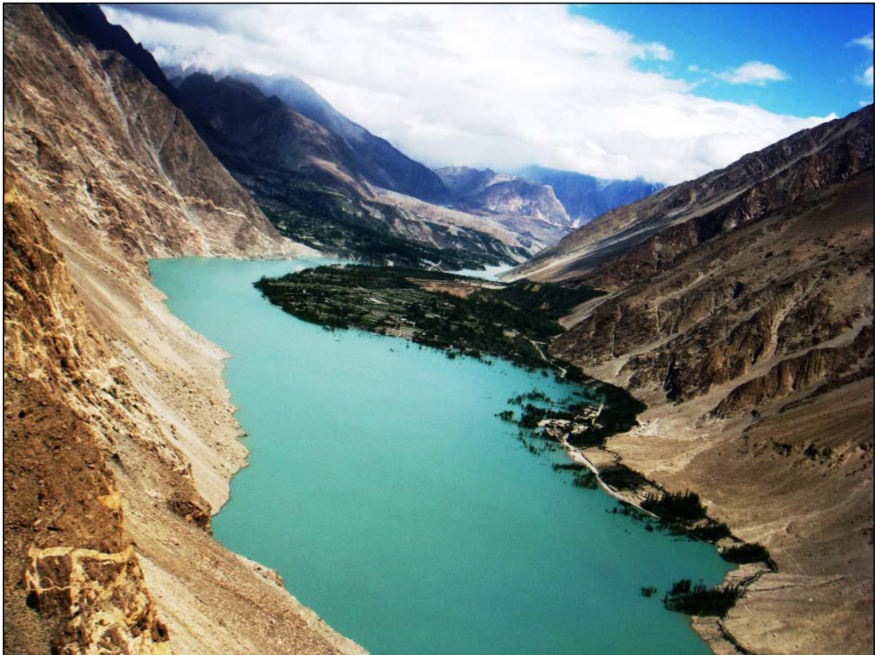
Figure 2.2: Aerial upstream view of 2010 Hunza landslide-dammed lake in northern Pakistan. This Pamir Times Photograph was taken on May 13, 2010 (127 day of impoundment) when lake waters constantly rising and filling the Hunza valley with pool height to be 2432 m.a.s.l. Another 12m increase was seen in lake prior to overtopping on May 29, 2010.
