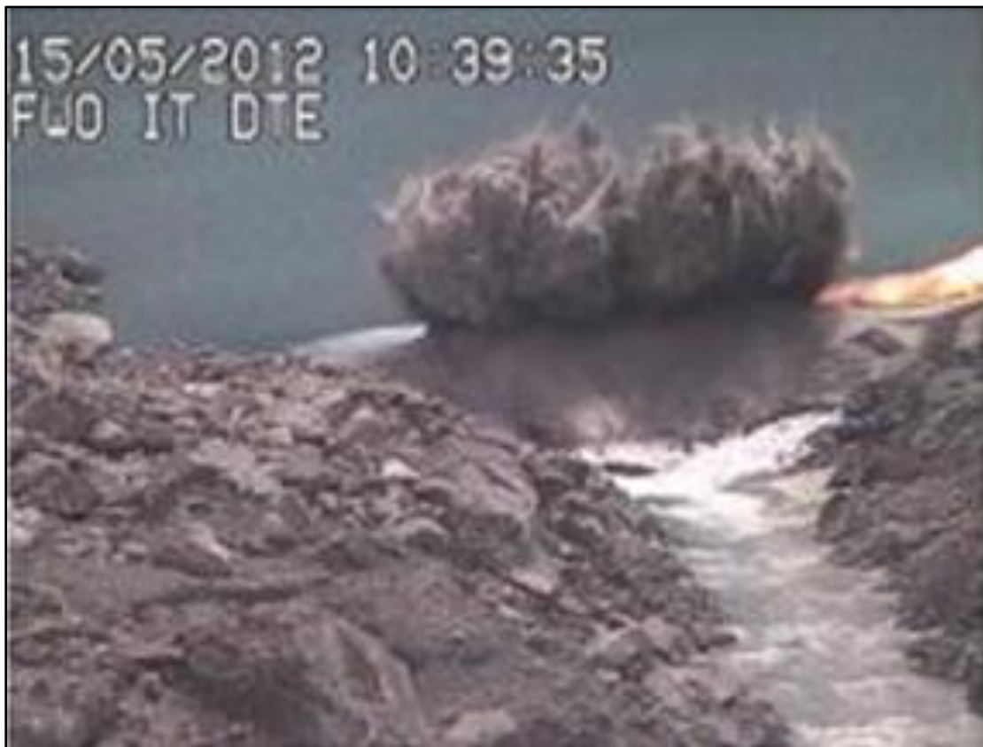
Figure 2.17: Snapshot provided by FWO on 15 MAY 2012 at the time of blasting of Attabad Lake Spillway.
