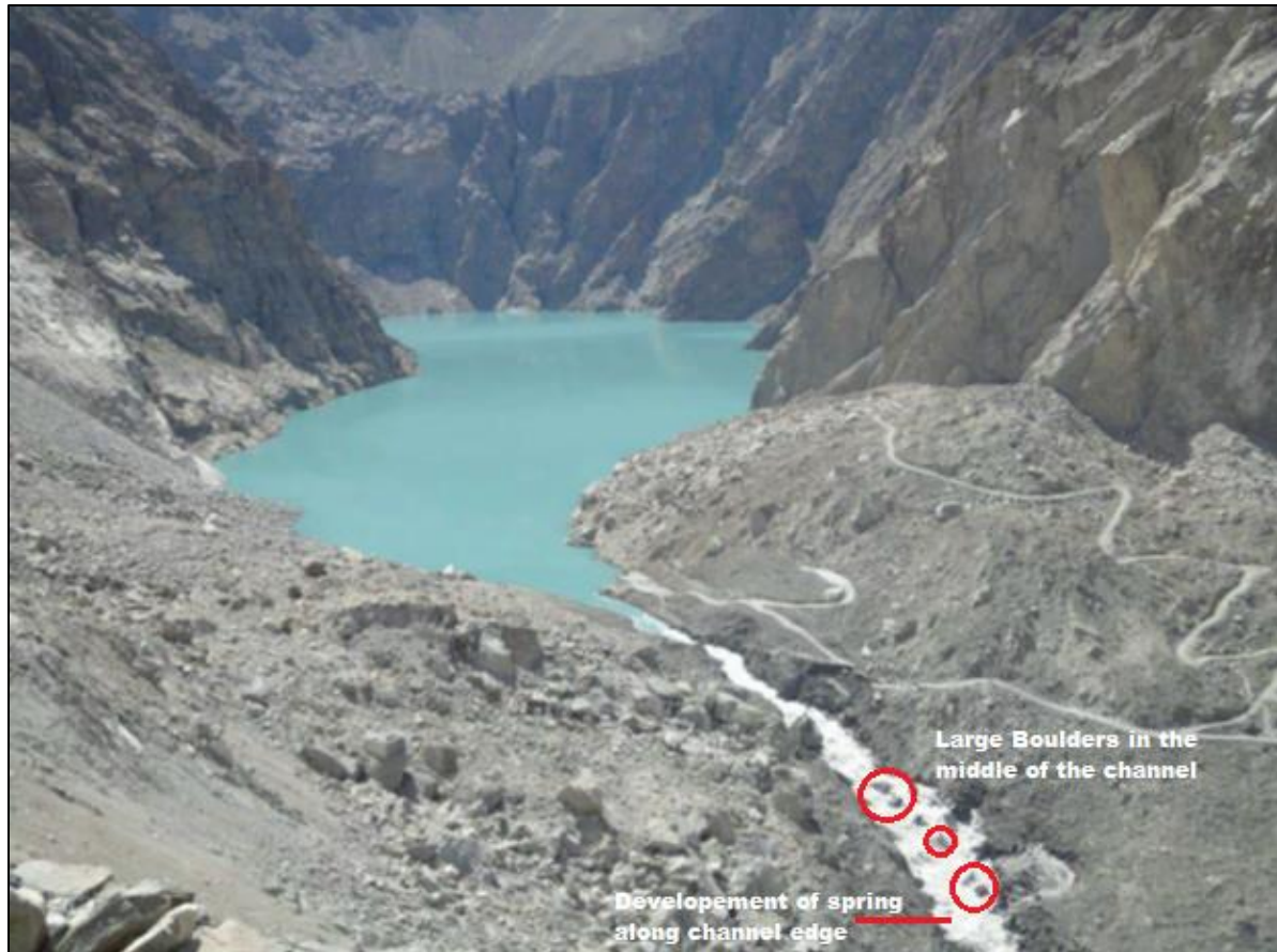
Figure 2.4: Photograph of Focus Humanitarian Assistance is taken on June 10, 2010 (12 days after overtopping), reveals flow along the spillway is prominently increased that controlled by the large boulder in the middle of the channel, also the deepening and the widening of the lower part of the channel with the formation of rapid is evident.
