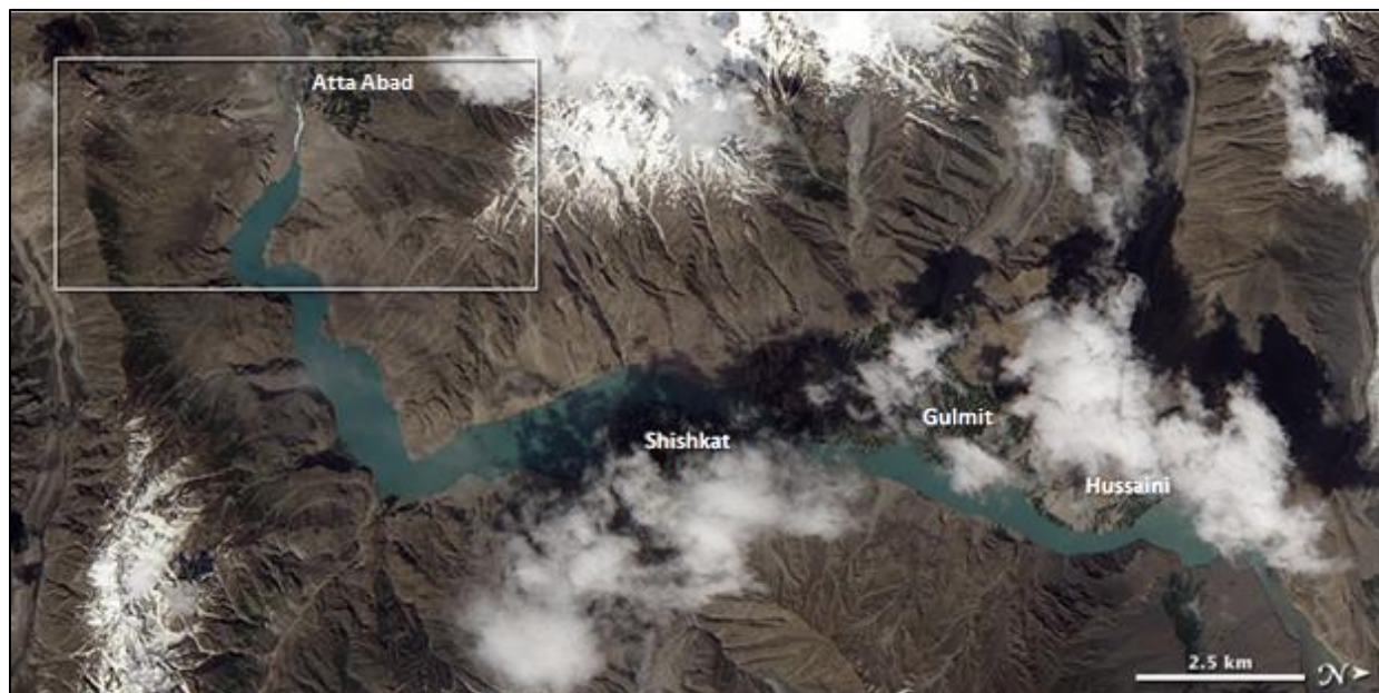
Figure 2.9: In this EO-1 satellite true color image, the lake appears to have overtopped the rocky dam on July 2, 2010 which backing up the waters of the river past the settlements of Shishkat, Gulmit, and Hussaini. Hunza River flows towards south in this rotated image in which north is at right.
