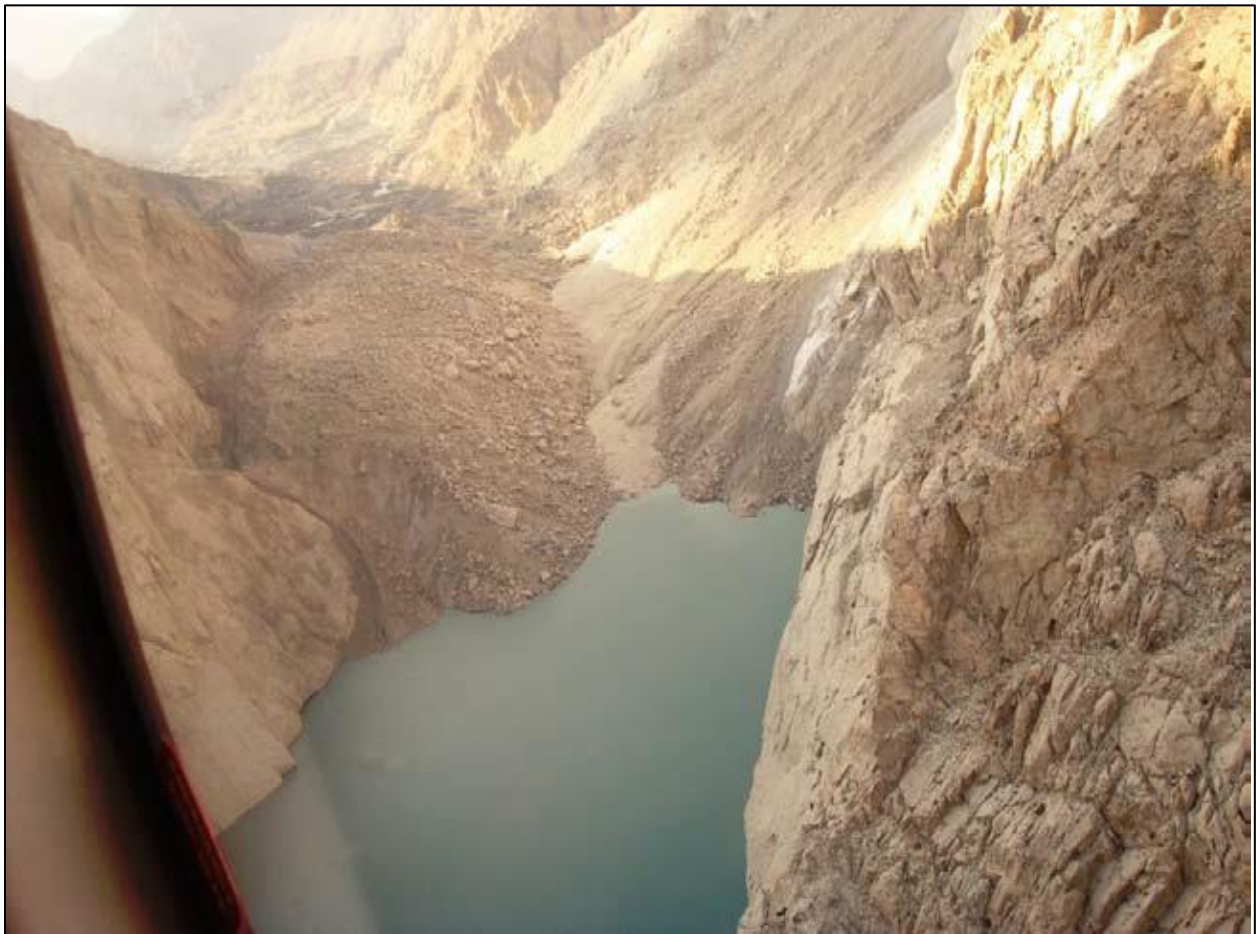
Figure 2.1: Aerial view of Attabad landslide (Viewing downstream) on January 17, 2010 (Day 13 of impoundment) and natural debris dam features also highlighted that blocked the Hunza River forming Attabad Lake, filling in lower foreground [Pamir Times photograph]
