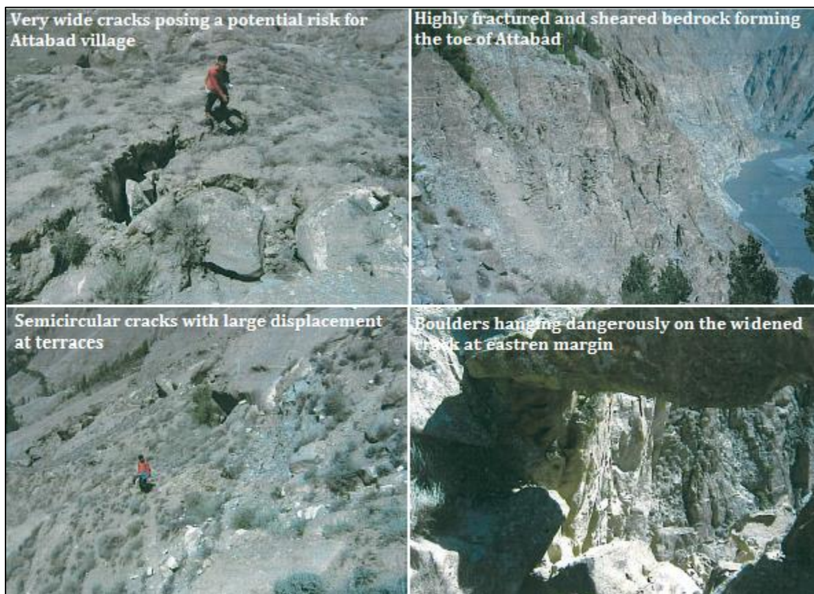
Figure 3.6: Types of cracks lying at different locations
