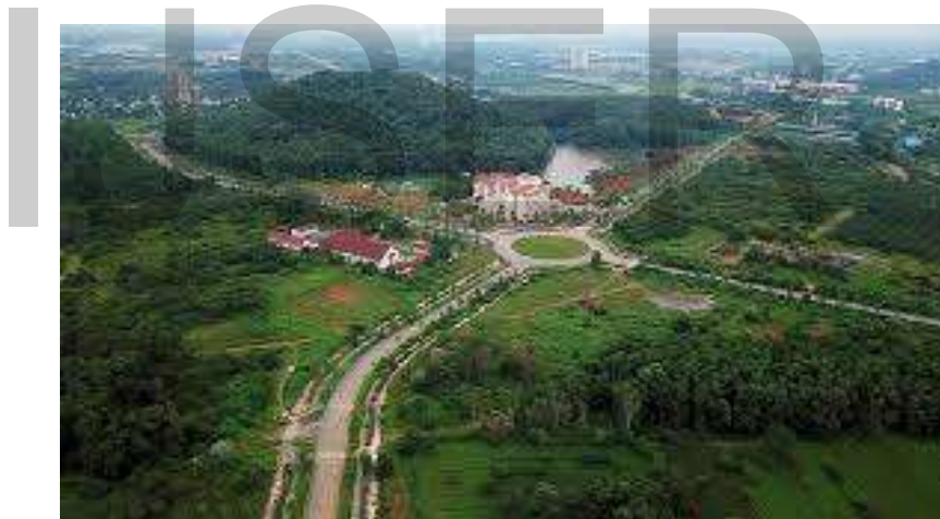
New Campus on the process of construction
