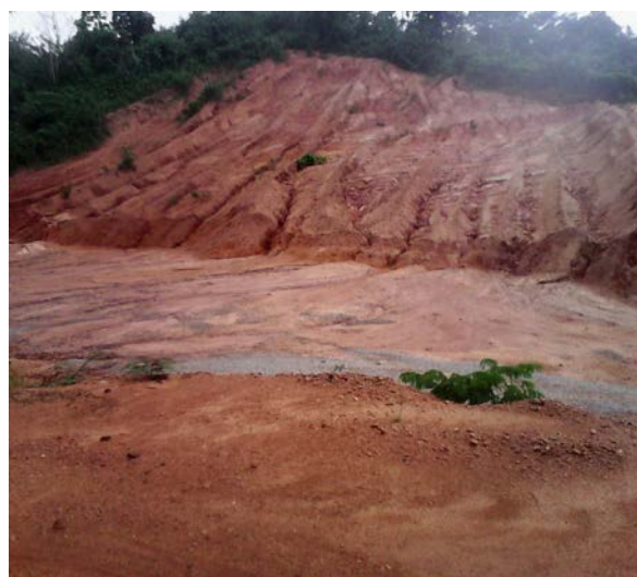
Fig. 2. The Plate showing the Project Site along Ikere-Igbara Odo Road, Ikere Ekiti, Ekiti State
