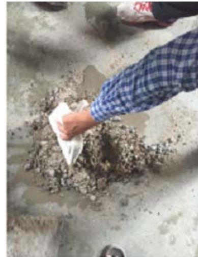
Fig. 4. Preparation of Concrete
