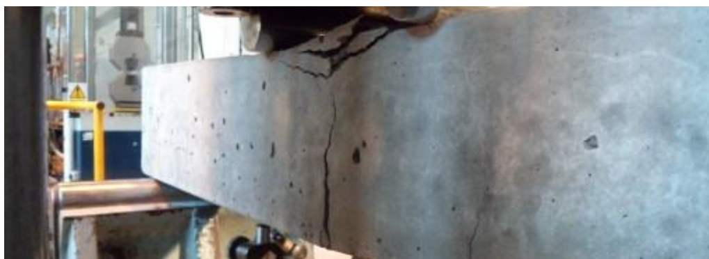
Fig 2: Flexural crack propagation of flexural series specimen
