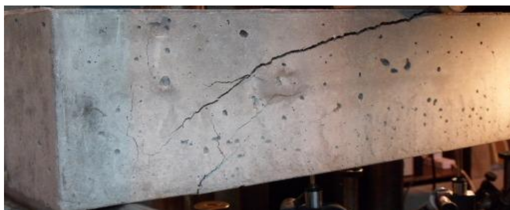
Fig 3: Critical diagonal crack propagation of shear series specimens
