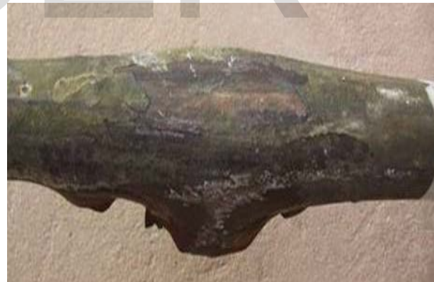
Figure 10. Photograph showing back view of the ruptured area of economizer tube and greenish deposits
