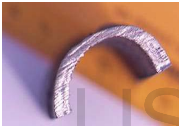
Figure 5. Photograph showing thinning of the tube wall of the economizer tube (side B)
