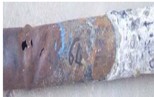
Figure 14. Photograph of the economizer tube B in as received condition showing (closer view)
