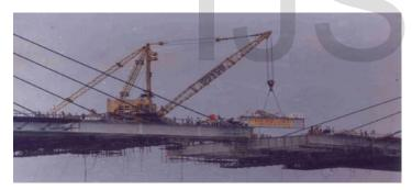
Figure 4. The mid-portion of the deck of the Second Hooghly Bridge being constructed, vividly showing some of the high capacity cranes used.
