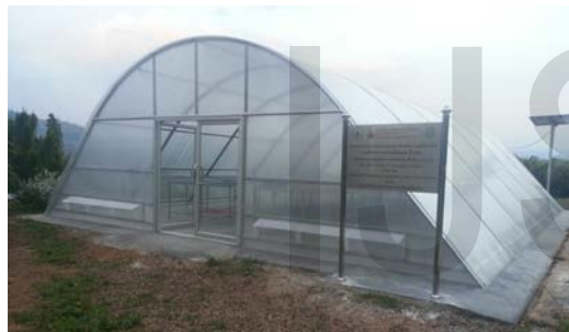
Fig. 1. The pictorial view of polycarbonate-covered greenhouse solar dryer, from the front side
